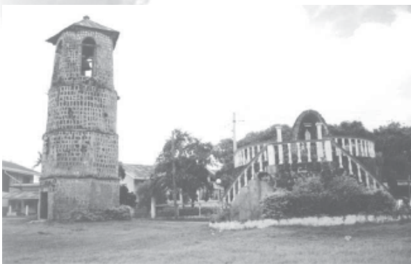
ST. FRANCIS DE ASSISI BELL TOWER - Poblacion, Siquijor. Siquijor - Built in 1870. From ground to roof, it is approximately 45 feet high . It is made up of stone formed into blocks called tablets.
